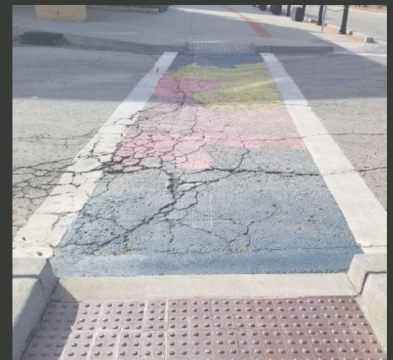
Mis-aligned ramp and crosswalk near McCoy Park
