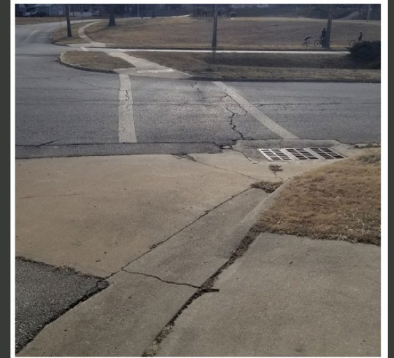
Mis-aligned ramp and crosswalk near McCoy Park
