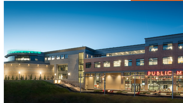
City of Lenexa, Kansas – Civic Center/ Recreation Center
