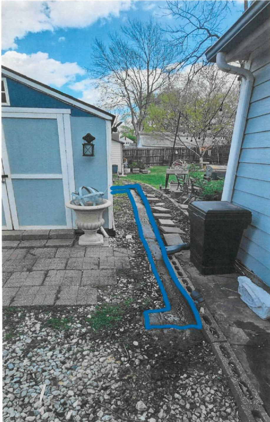
Upclose of footing and old shed.
