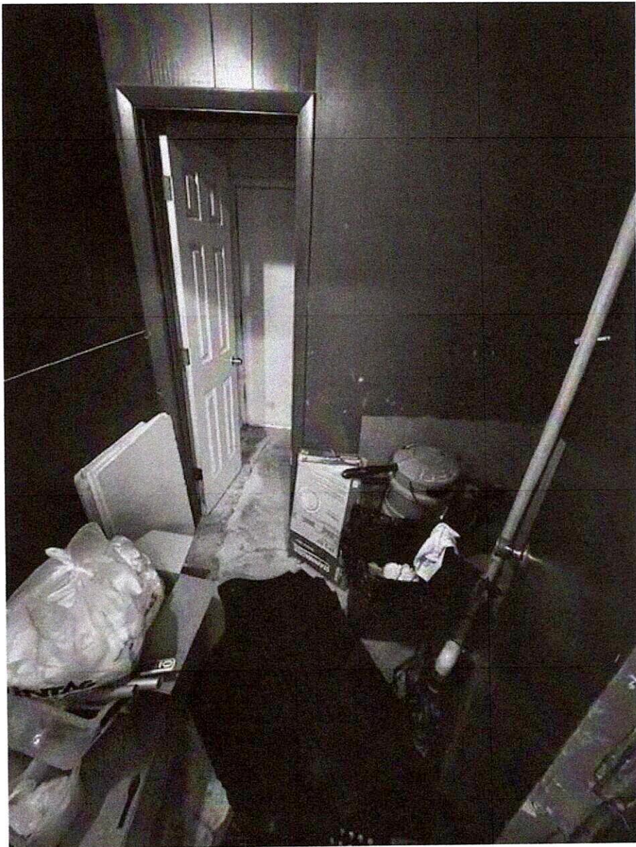
Grease Trap / Sump Pump
