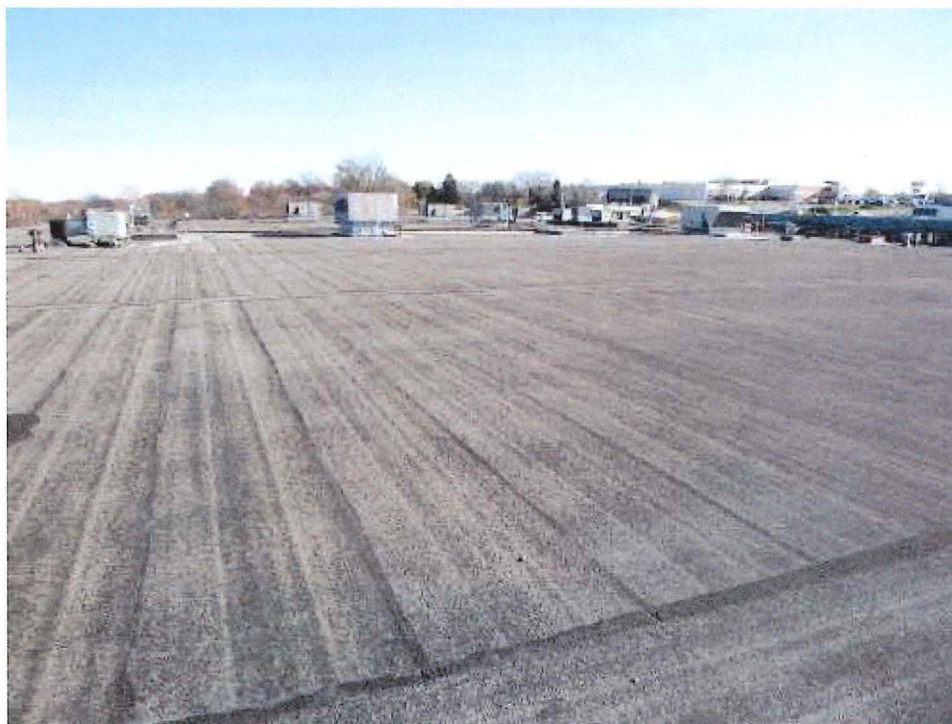
4466 S Noland Rd – built up roof with mineral cap sheet
