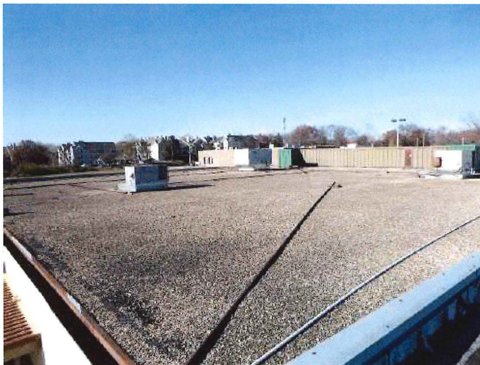
4452 and 4460 S Noland Rd – built up with embedded gravel ballast
