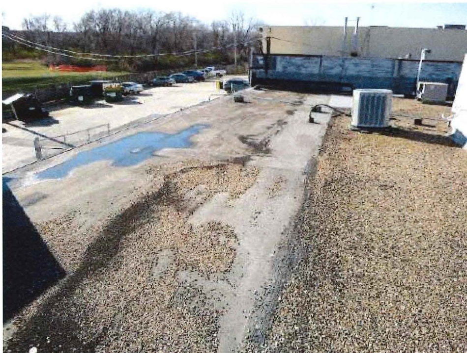
4486 S Noland Rd – patching of roof
