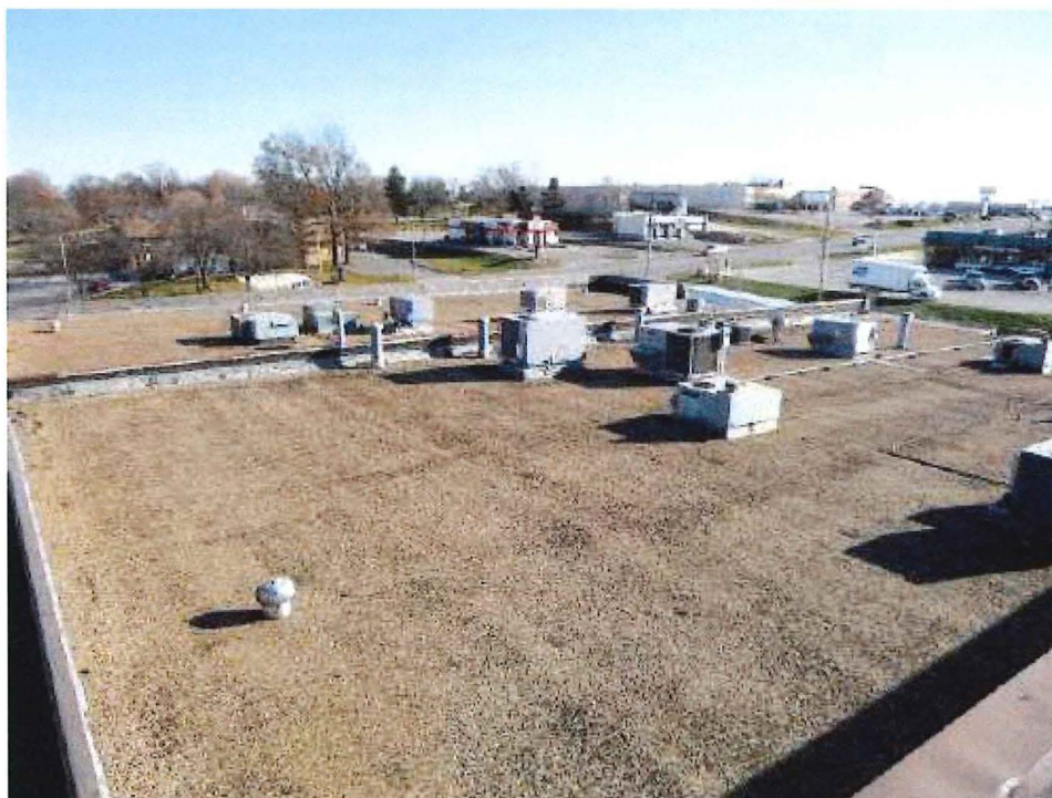
4480 S Noland Rd – built up roof with embedded gravel ballast
