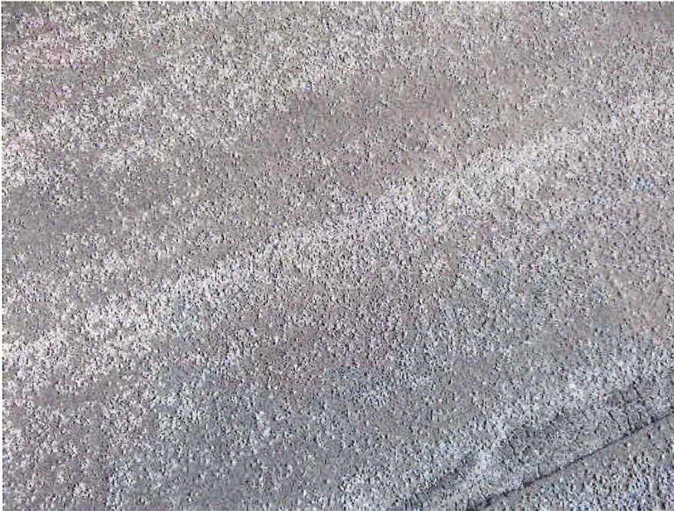
4466 S Noland Rd – mineral cap sheet extremely worn
