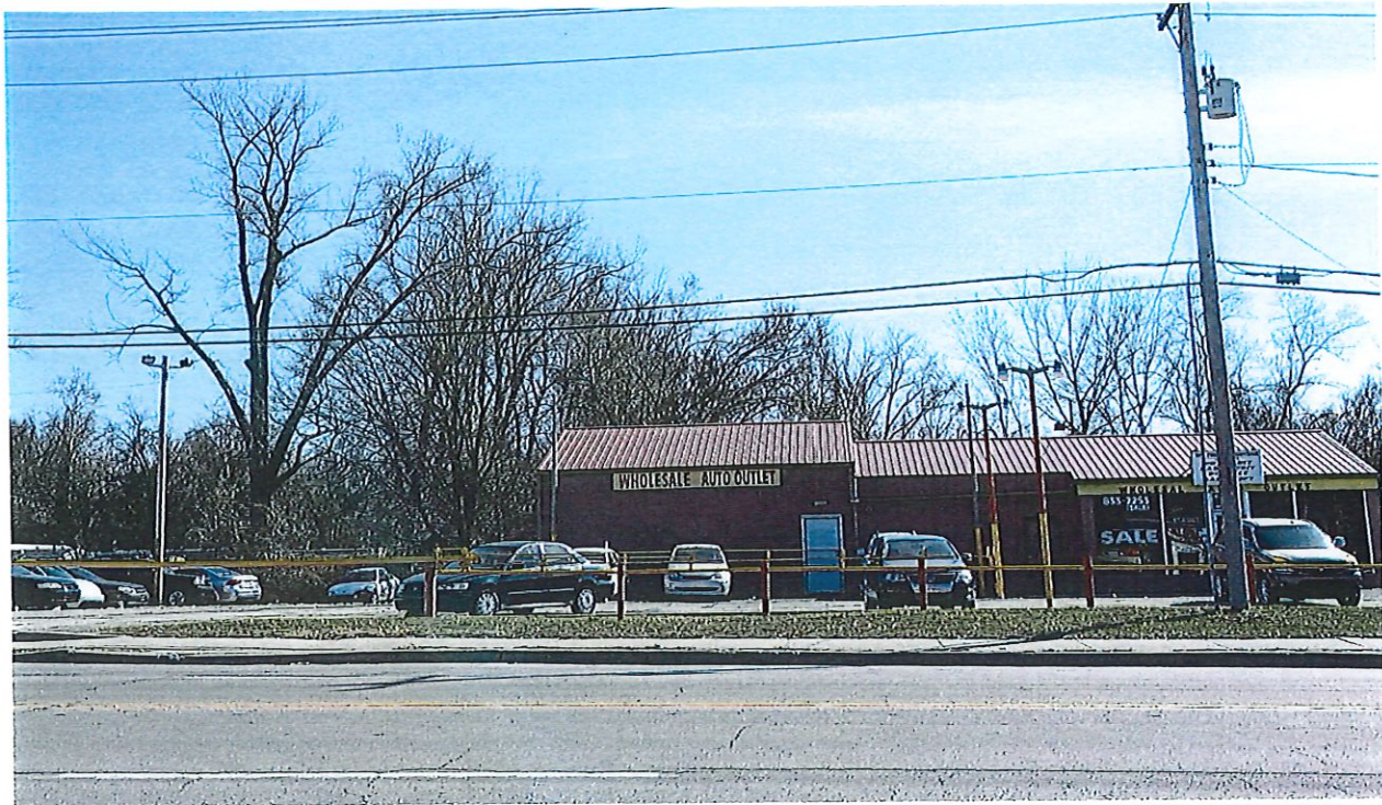
Parcel No.27-120-01-17-00-0-00-000 Curbing is deteriorating.
