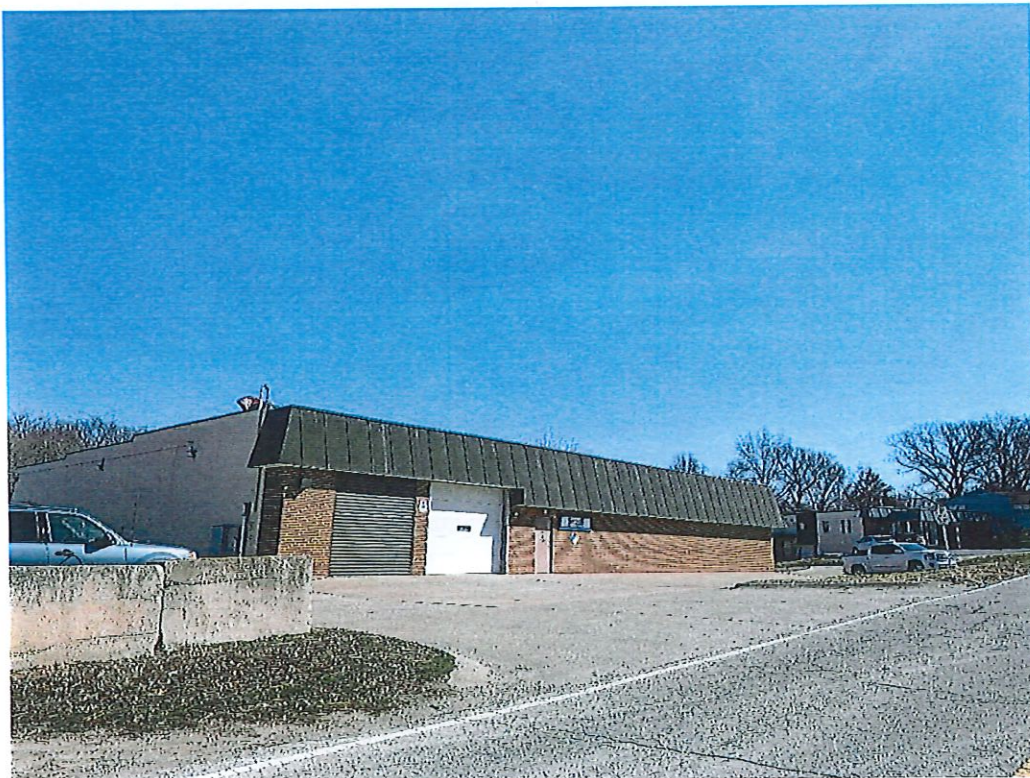
Parcel No. 27-120-18-01-00-0-00-000 No sidewalks.
