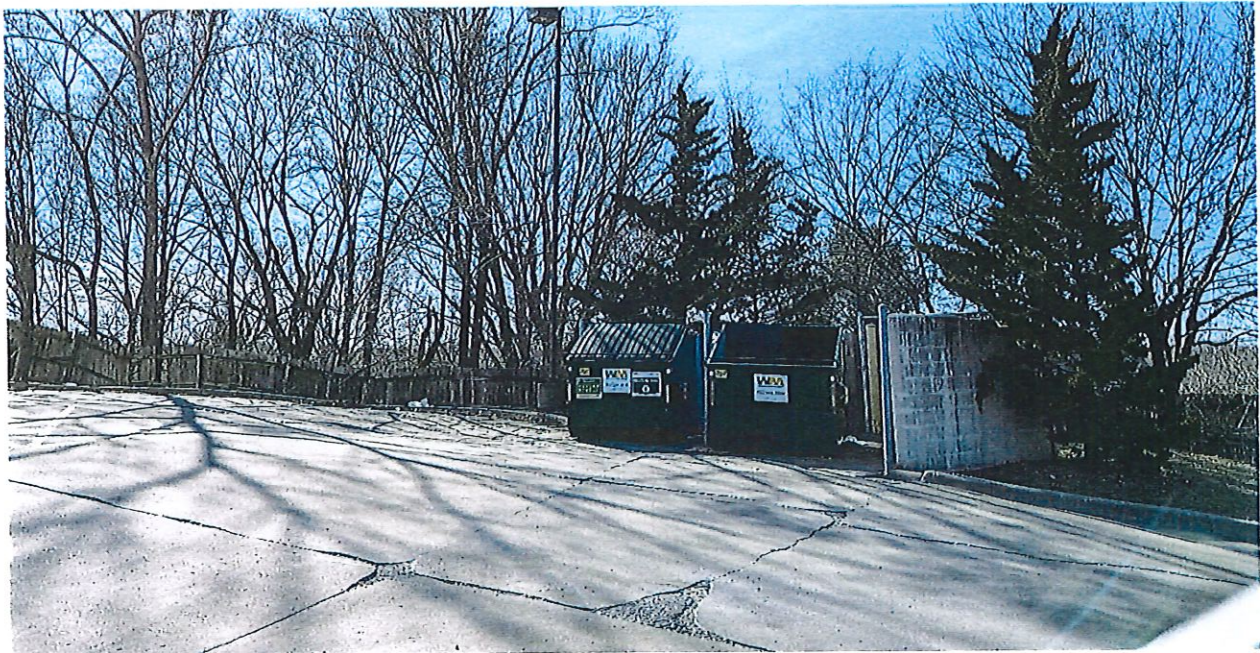
Parcel No. 27-110-04-42-00-0-00-000 Poor conditions of parking lot. Broken fence.
