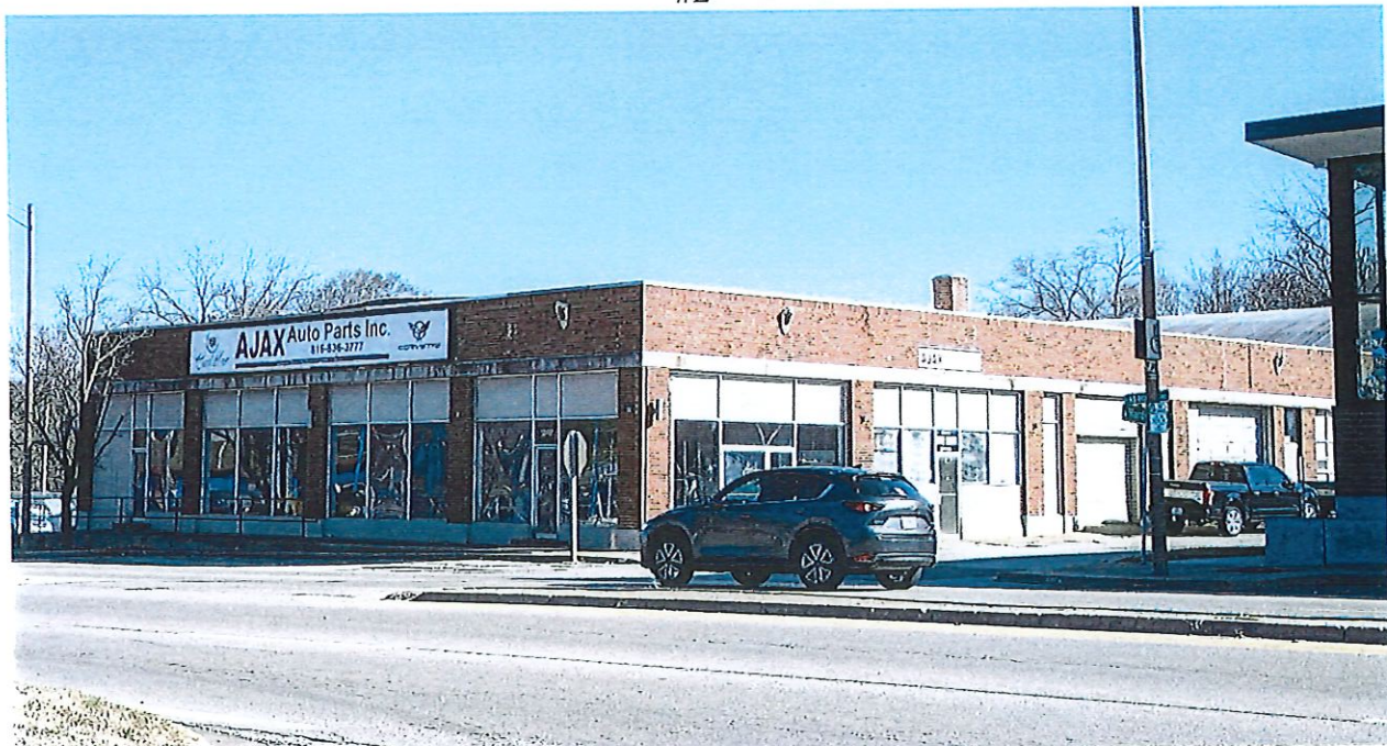
Parcel No. 27-120-06-77-00-0-00-000 Façade in need of improvement. #2
