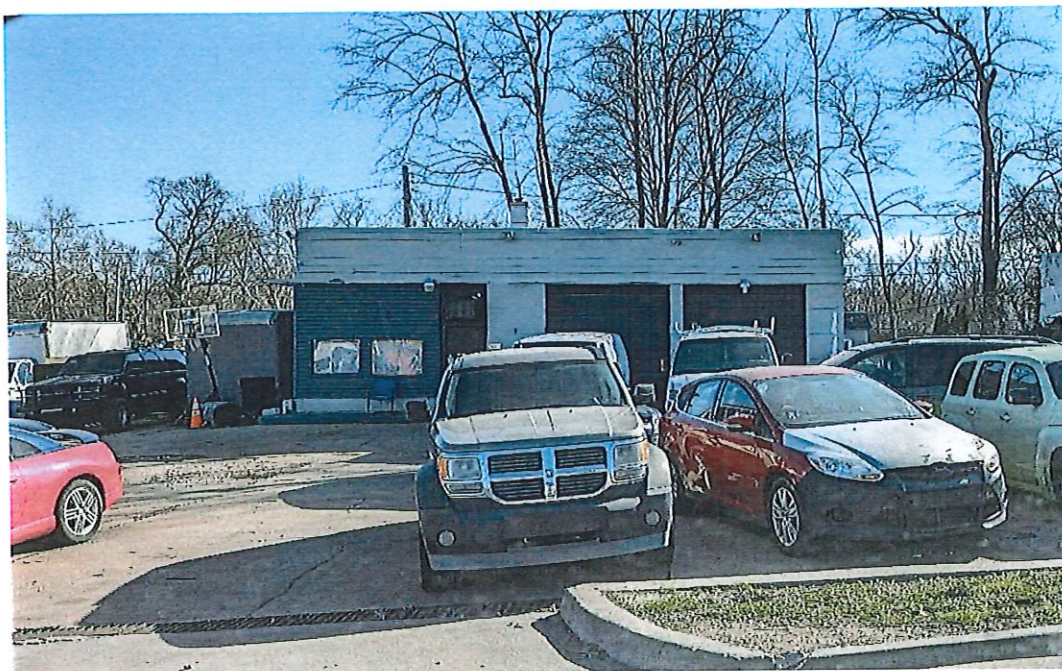
Parcel No. 27-120-02-02-00-0-00-000 Poor condition of parking lot. Broken cars.
