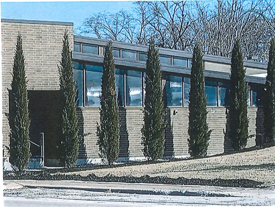
Parcel No. 27-120-07-36-00-0-00-000 Curbing in need of replacement.
