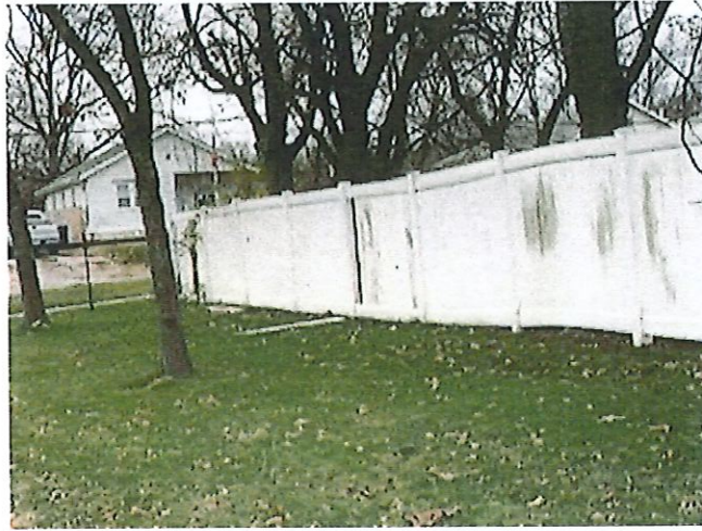
Parcel No. 26-320-05-41-00-0-00-000 Fence in disrepair
