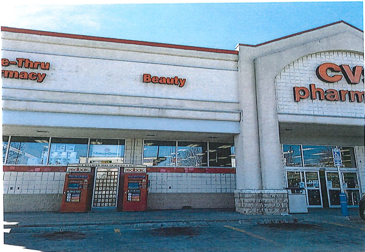
Parcel No. 27-110-04-42-00-0-00-000 Façade in need of improvement.
