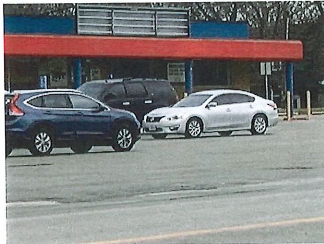
Parcel No. 15-940-10-00-0-00-000 Broken storefront sign
