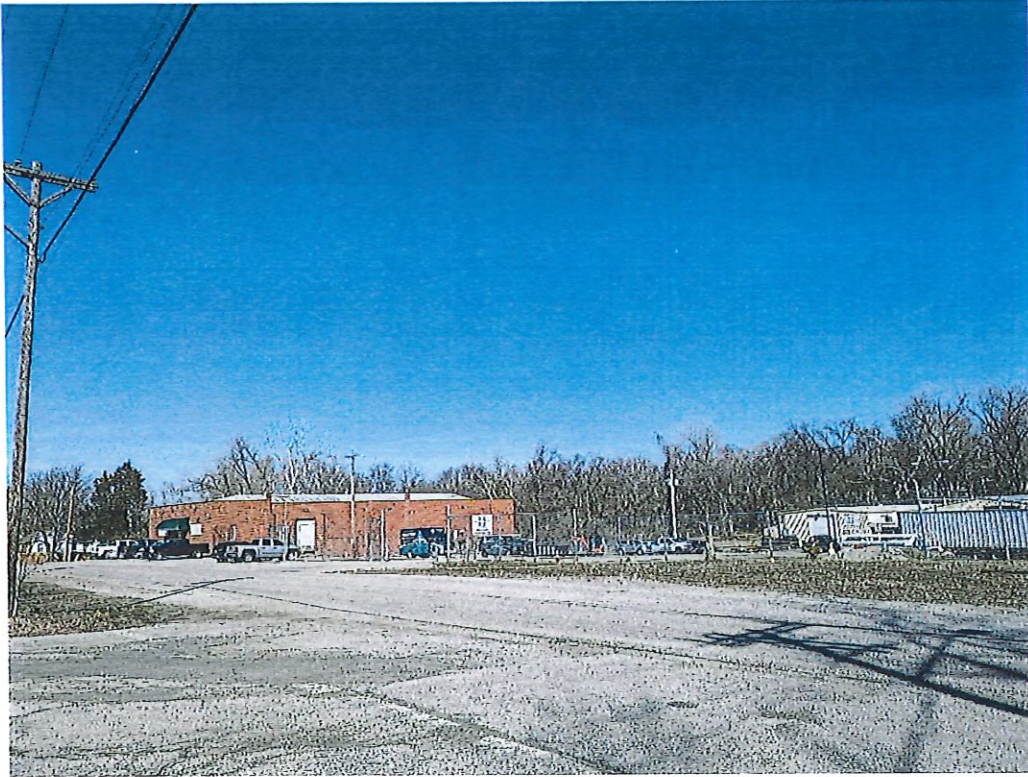
Parcel No. 27-120-17-02-00-0-00-000 No sidewalks
