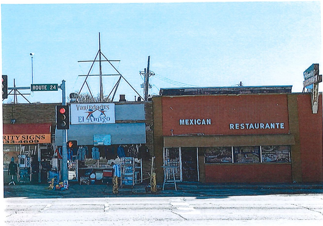
Parcel No. 27-120-08-33-00-0-00-000 Curbing in disrepair. #2
