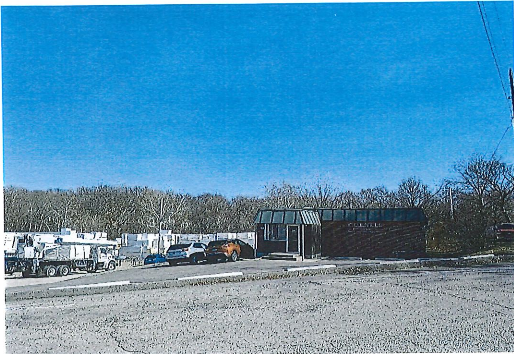
Parcel No. 27-120-18-01-00-0-00-000 No sidewalks. #2
