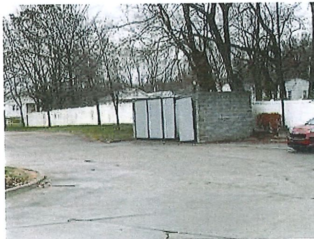
Parcel No. 27-110-01-02-00-0-00-000 Trash enclosure in disrepair
