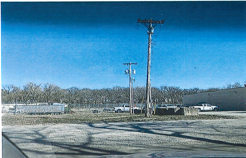
Parcel No. 27-120-18-01-00-0-00-000 No sidewalks.
