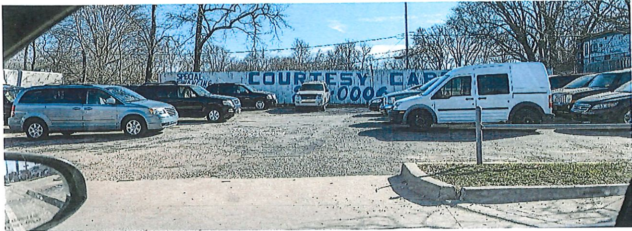
Parcel No. 27-120-02-05-00-0-00-000 Fence in need of improvement. Parking lot and curbing in need of repair.
