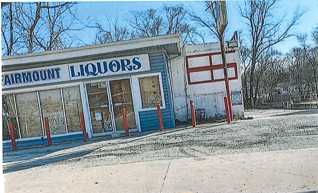
Parcel No. 27-120-01-24-00-0-00-000 Poor condition of parking lot. Boarded up building.
