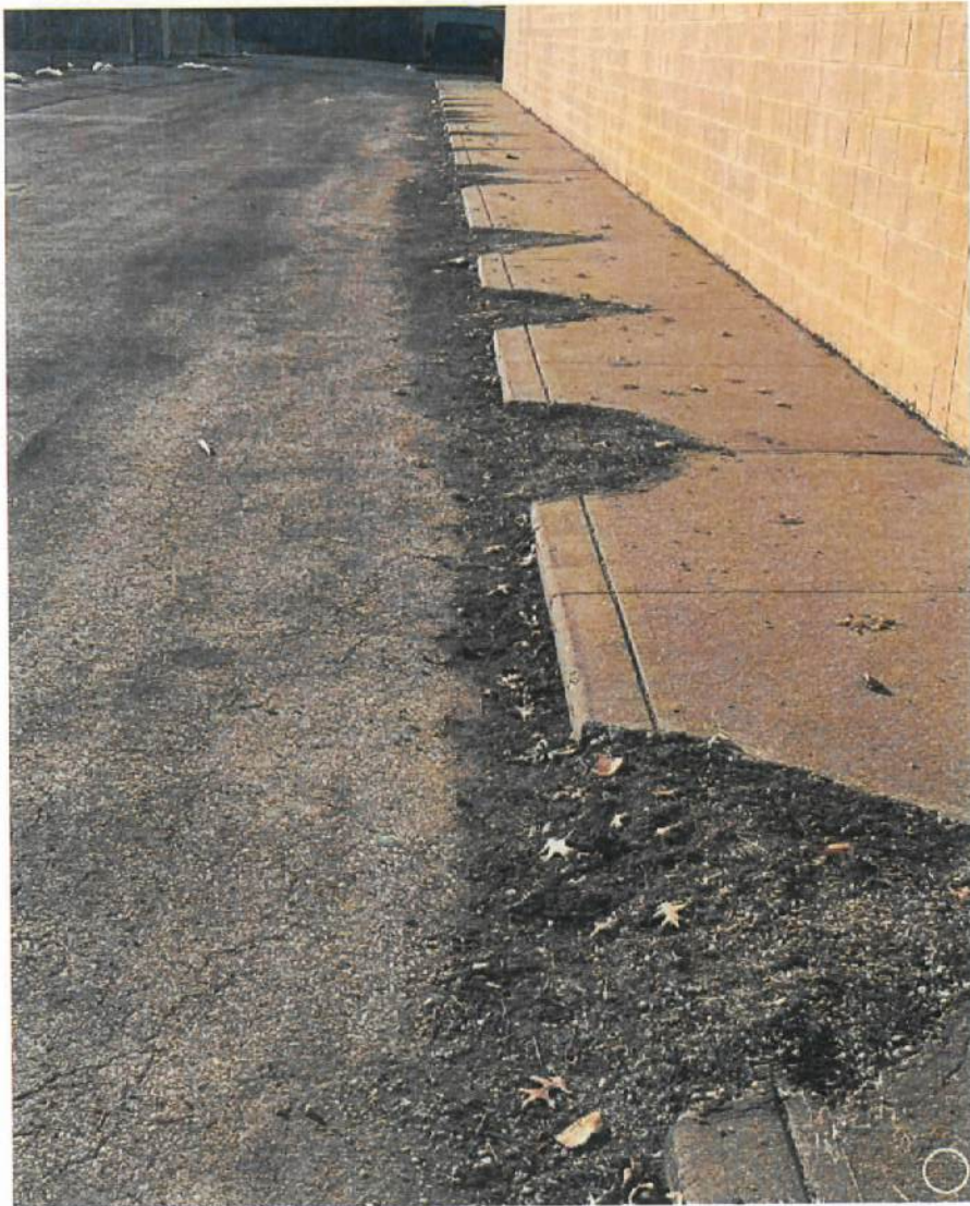
Deteriorated Sidewalk
