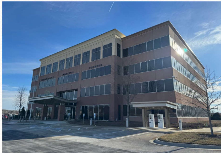
Front Entrance and Kiosks
