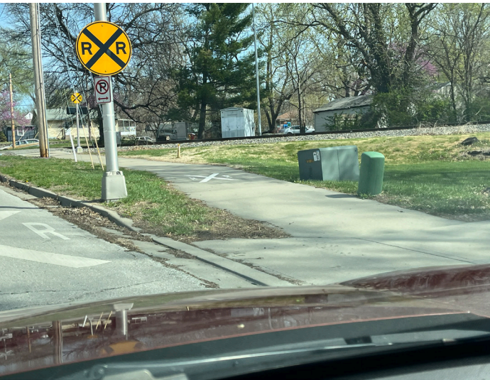
Railroad crossing for street and trail.
