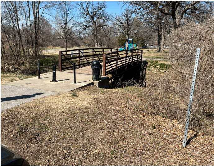
Entry bridge from parking lot.
