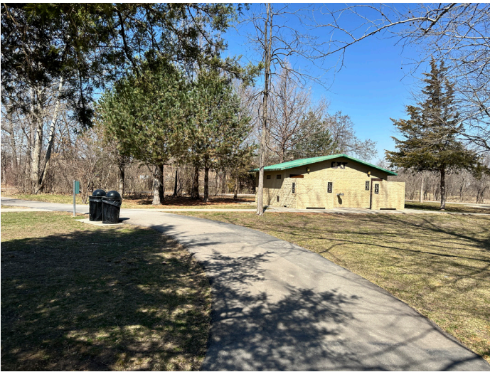
Restroom facility near the parking lot and playground.
