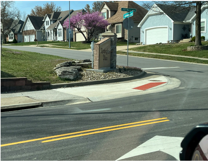
Refurbished crosswalk corner.
