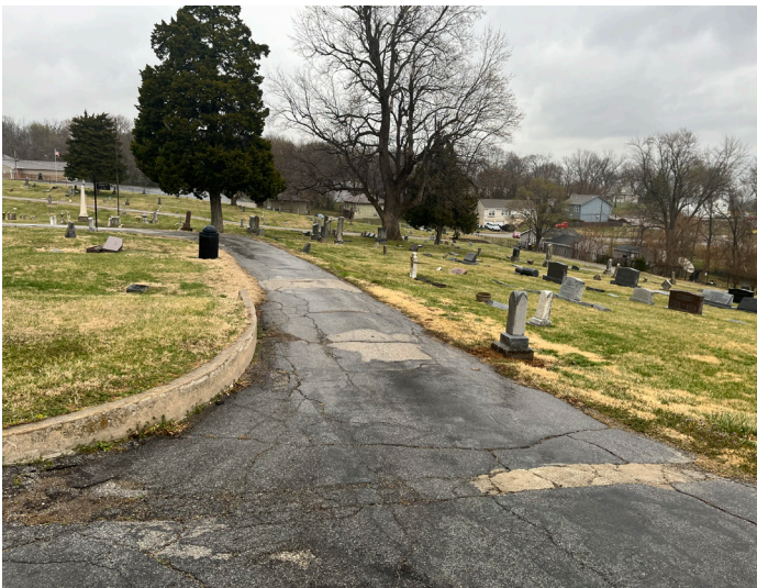
Road and curb near headstones.
