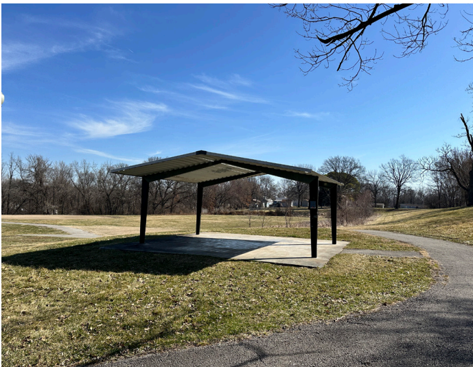
Park shade structure connected by path.
