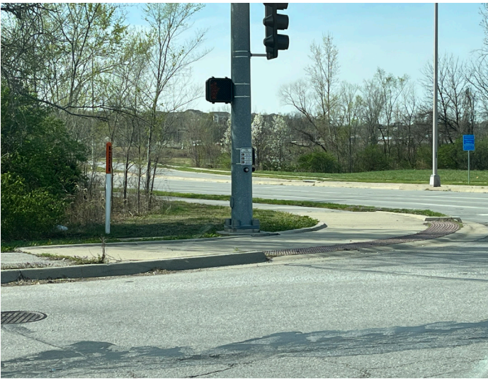
Intersection has pedestrian signals and crosswalks.
