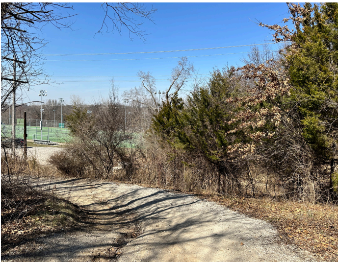
Trail shows signs of erosion in some places and makes for an uneven surface.
