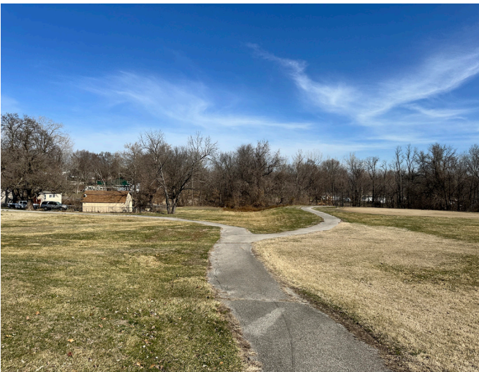
Park walkways (asphalt material).
