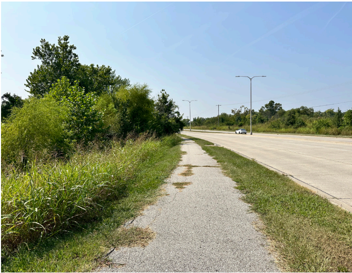
Asphalt paving along the trail.
