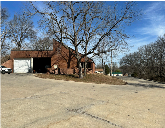
Parking area behind fire station.
