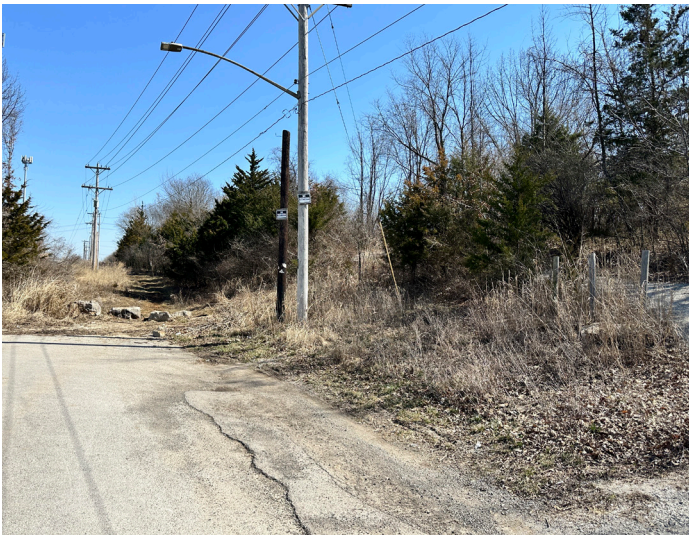
Entry drive has no signage near secondary trail entrance.
