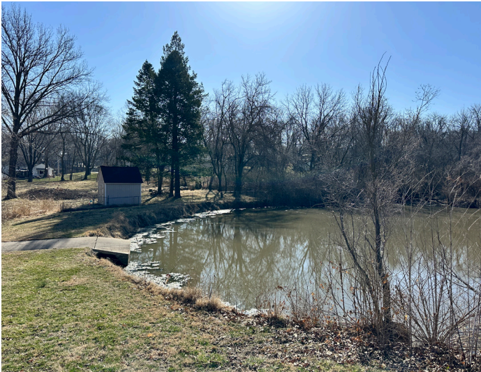
Concrete channel directed into the pond.
