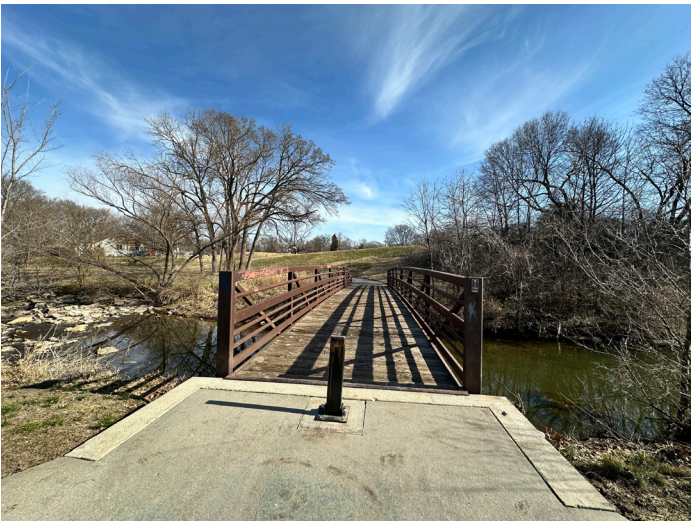
Bridge across small creek into other half of the park.
