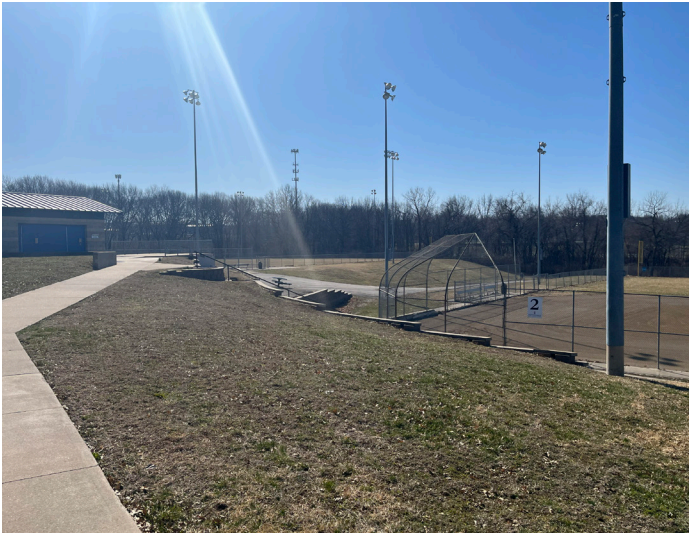
Sidewalks and trails have elevation changes in the practice field location.
