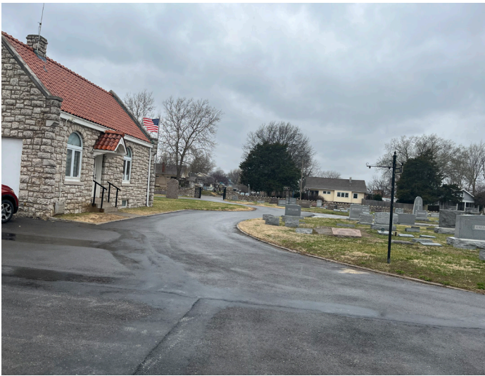
Sexton Office near entrance.
