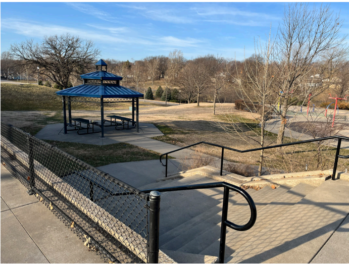
Terraced portions of the park with easy to access stairs and ramps.
