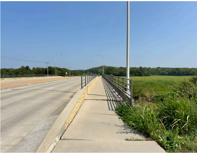
Bridge condition along 39th.
