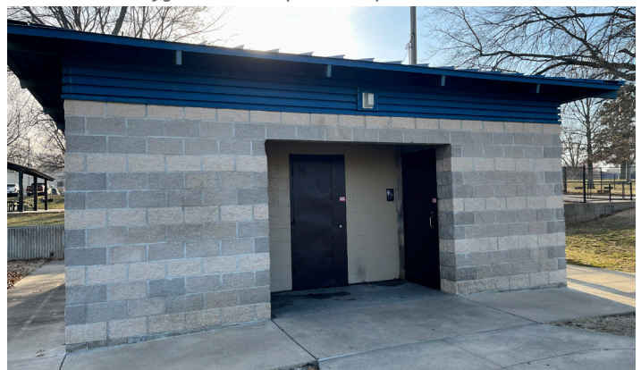
FIGURE 1.4 - Restroom at McCoy Park
