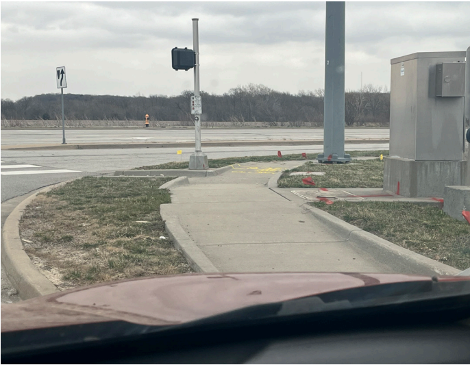
Sidewalk at crosswalk.
