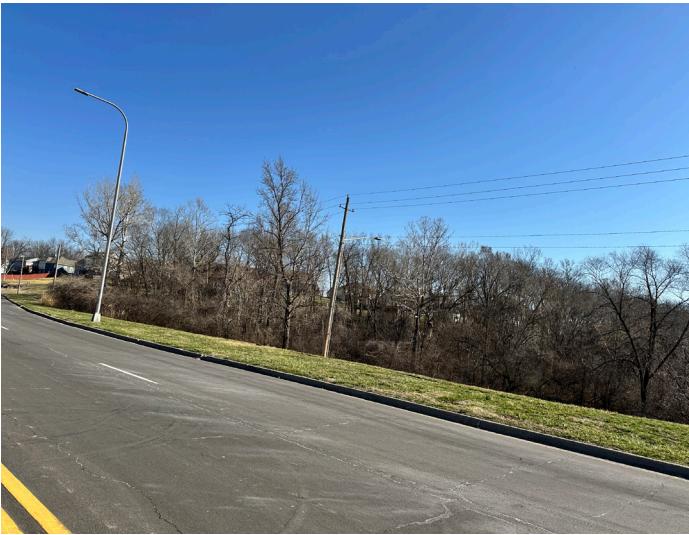
No sidewalk or on-street parking stalls, makes access difficult.
