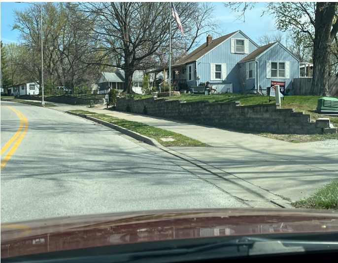
Portions of trail have retaining walls.
