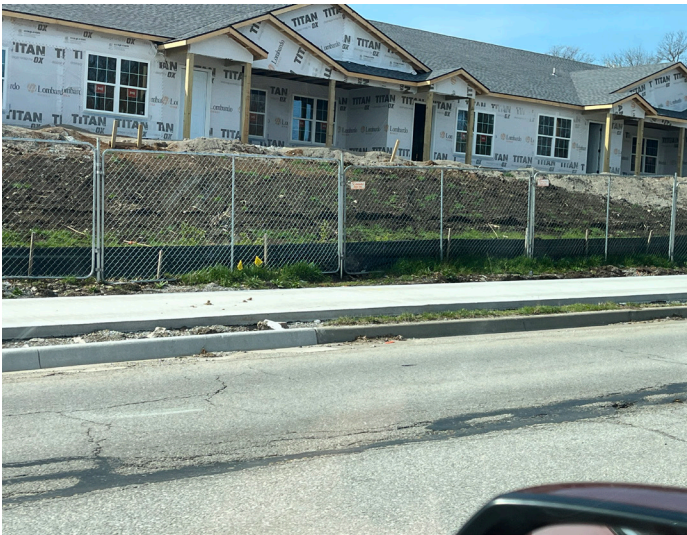
Some stretches of trails are newly poured concrete.
