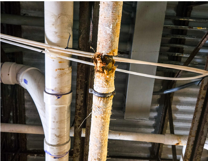
Damaged piping.
