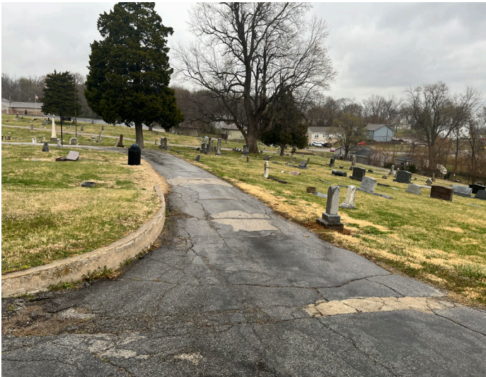
Road and curb near headstones.
