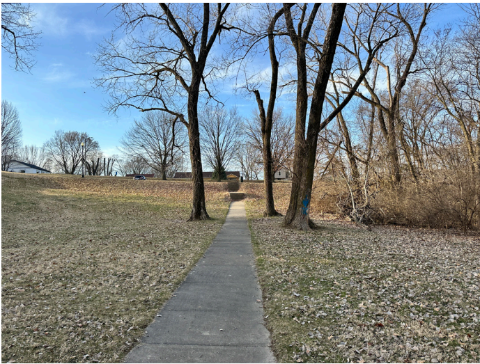
Stairs and sidewalk leading to parking lot.
