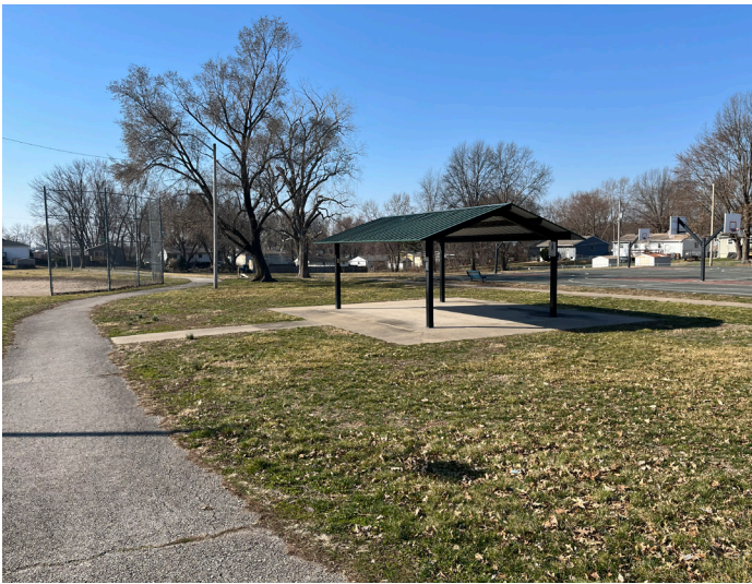
Shade structure located near the baseball field and basketball courts.
