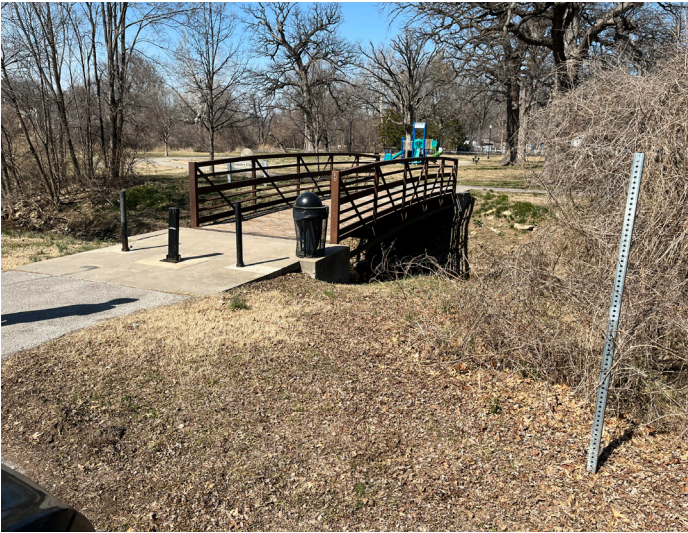
Entry bridge from parking lot.
