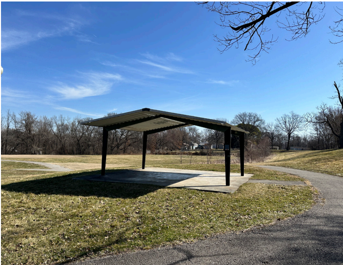
Park shade structure connected by path.
