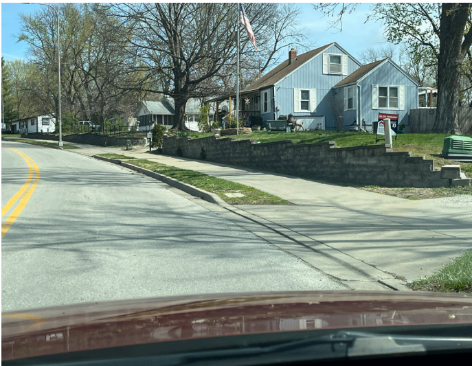
Portions of trail have retaining walls.
