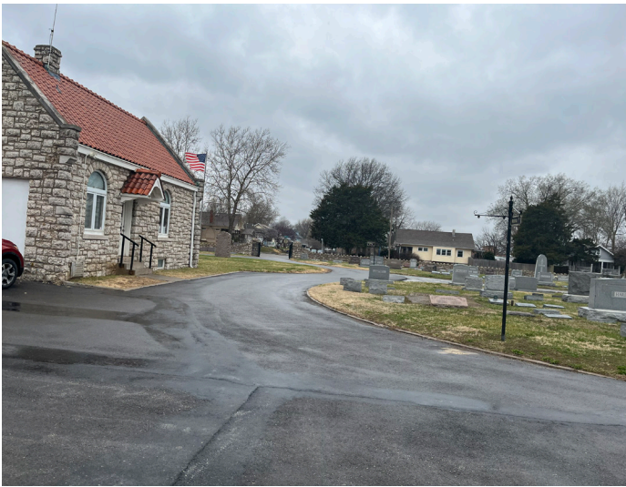
Sexton Office near entrance.
