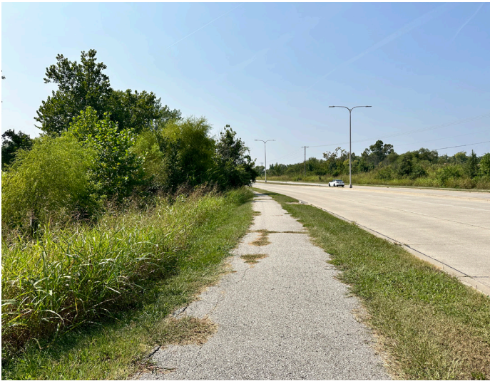
Asphalt paving along the trail.
