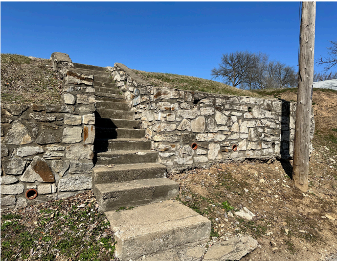
Stairway up to open lawn.
