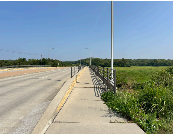
Bridge condition along 39th.
