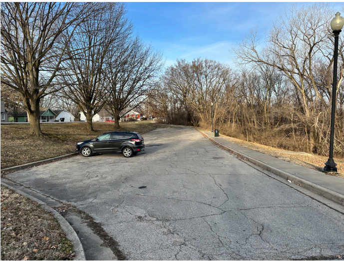
Parking lot lacking parking stripes.
