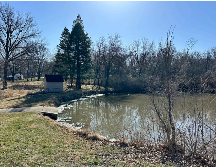
Concrete channel directed into the pond.
