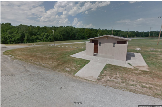
Restroom facilities seen on Google street view. (Permanently Closed)
