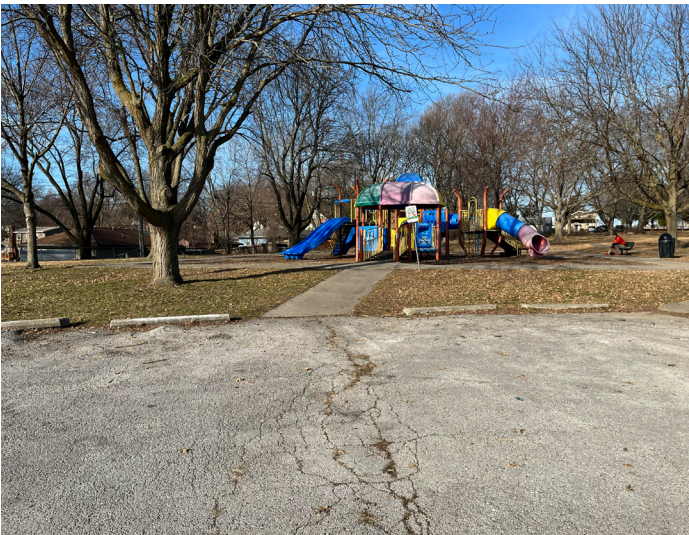
Additional playground structure.
