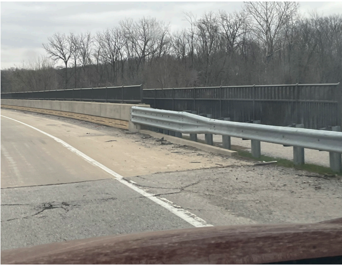
Trail extends across a bridge with barriers between street and trail.
