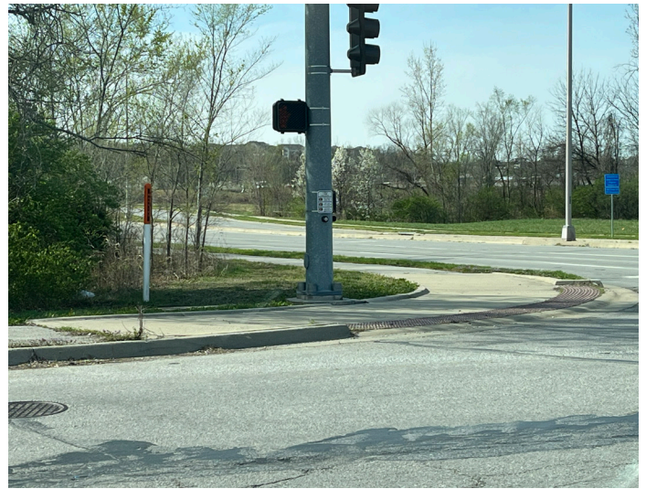
Intersection has pedestrian signals and crosswalks.
