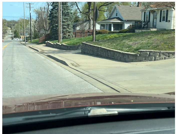
Portion of trail with no planted median.
