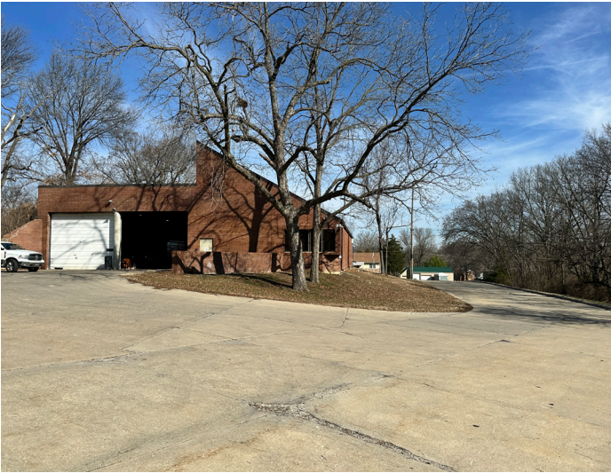
Parking area behind fire station.
