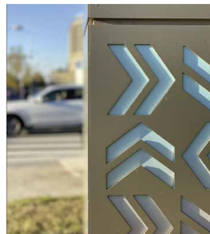
DIFFUSED, ILLUMINATED ACRYLIC ACRYLIC WITHIN SIGN CABINET, FLUSH-MOUNT TO FACE
