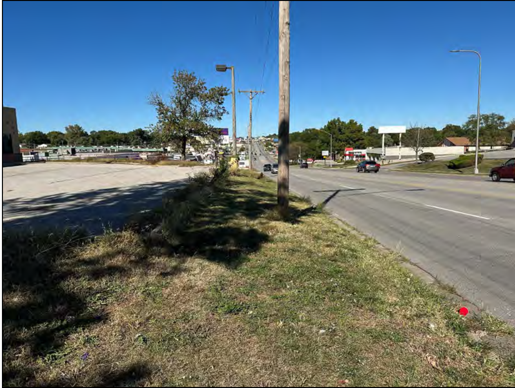
Lack of sidewalk
