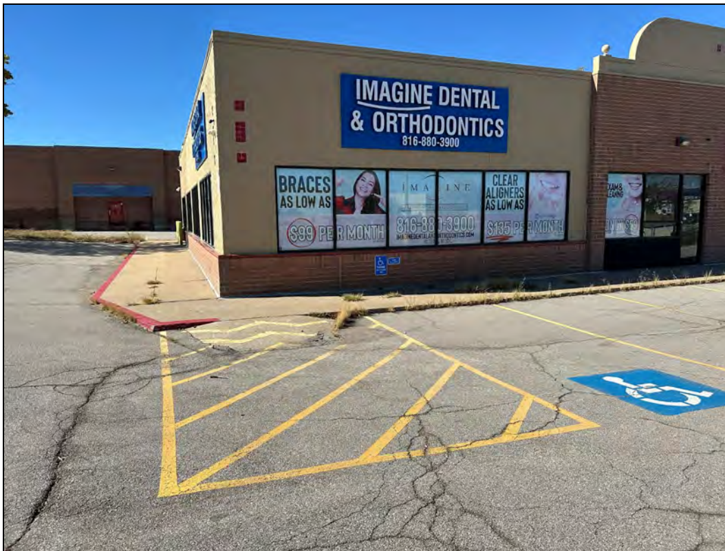
ADA Signage and ramp not code compliant
